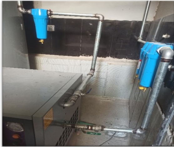
Sorting Machine – At a MG Beneficiary Site
